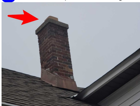
Flue cap missing
