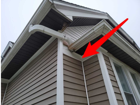
Missing downspout
