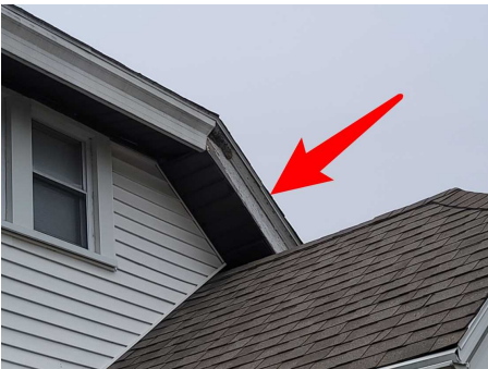
Missing flashing
